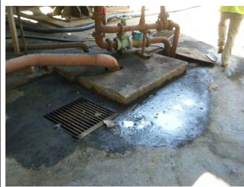
Photo 6. Oil staining from spill in April 2011, adjacent to location SB13.
