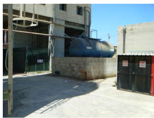
Photo 5. Bunded gas oil tank
