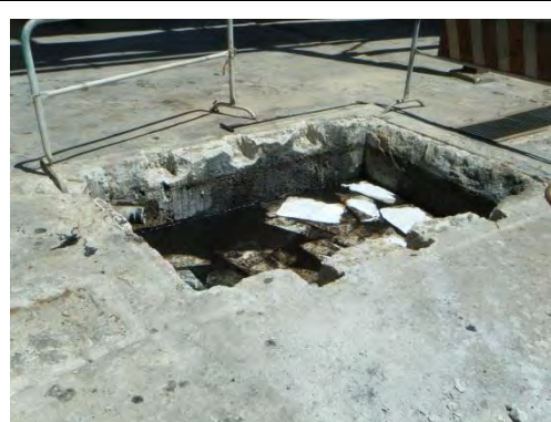
Photo 3. Oil interceptor adjacent to SB07
